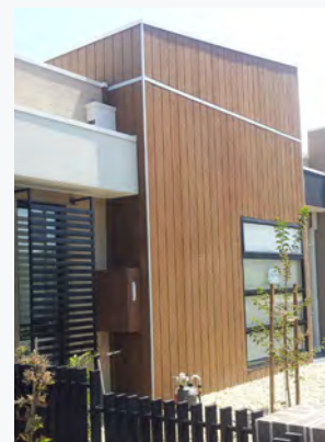
4 MONTHS: The board shows signs of lightening.
