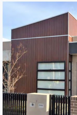
COMPLETE: After 3 coats the timber is restored and is now UV protected. Maintain the stain over time as per product directions to continue to protect the timber from UV rays.
