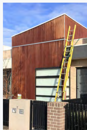
CLEANING: Wash the boards with a product like Intergrain Reviver or Cabots Deck Clean and a firm brush.
